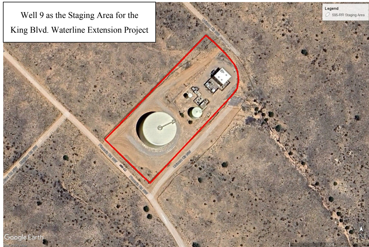
Figure 5. Close-up of Well 9, depicting the proposed Staging Area (red outline)
